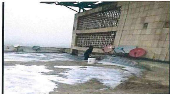
Step4:- Absorption coat applied for proper bonding of Thermacool
