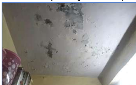
Condition of Apartment Rooms
