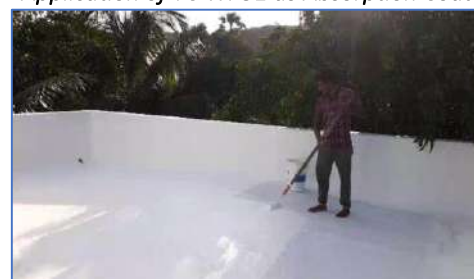
Application of 2 Coats of TC 0.3C
