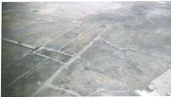
Step3: - Application of WP51+Cement coat to fill the crakes in concrete
