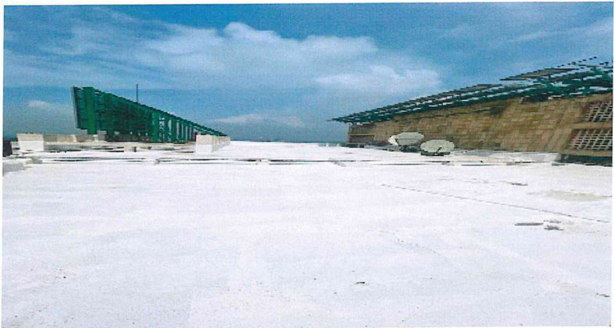
Roof after final coat of paint
