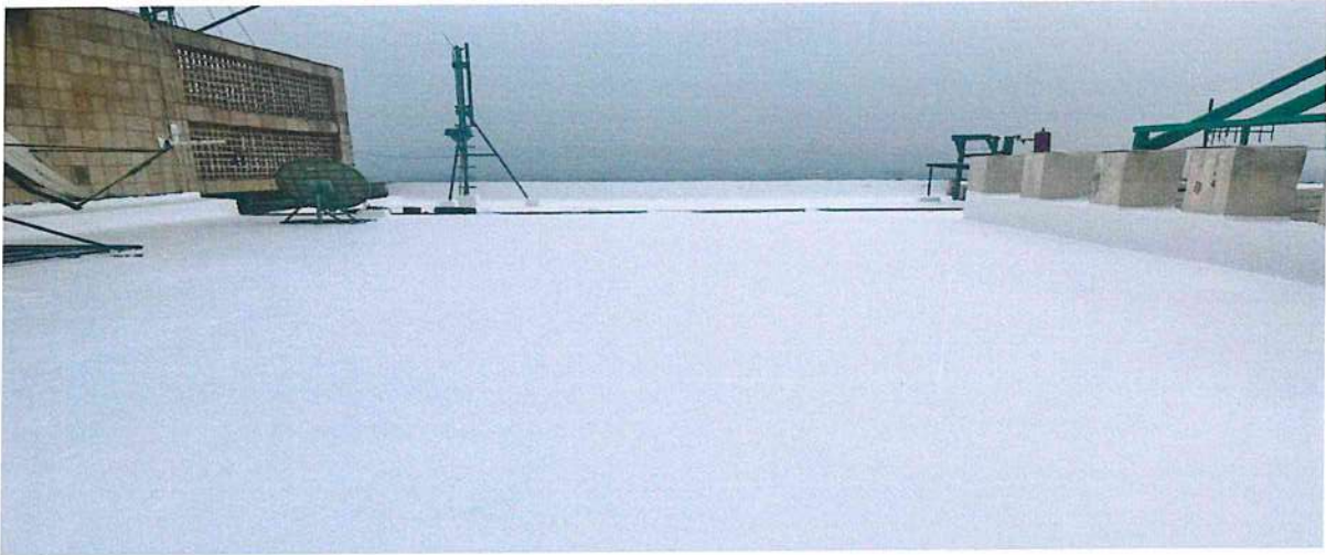
Step5: - Application of first coat of 0.3C Thermacool paint
