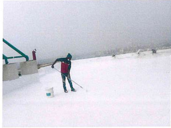
Step6:- Application of second coat of Thermacool paint
