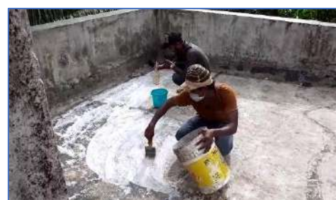
Application of TC WP51 as Absorption Coat
