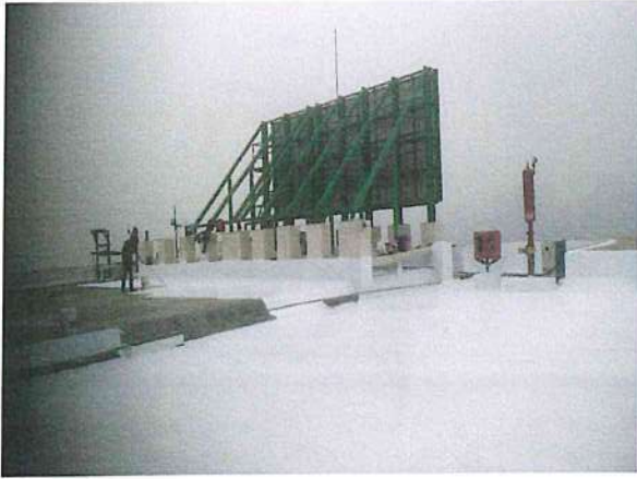
Step5: - Application of first coat of 0.3C Thermacool paint
