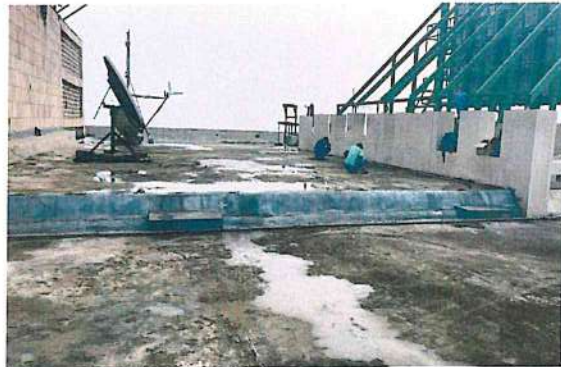
Step2:- Brooming of surface to identify the crake
