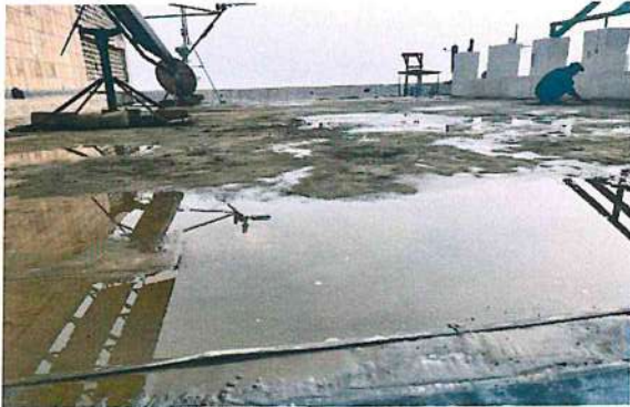
Step1: - Cleaning of roof with water
