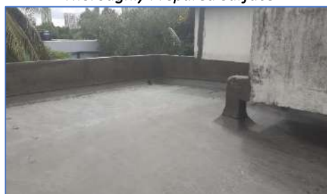
TC WP51 Waterproofing 2 Coat Applied
